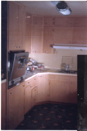
1960's New kitchen, Marstellar House, College Station, TX
